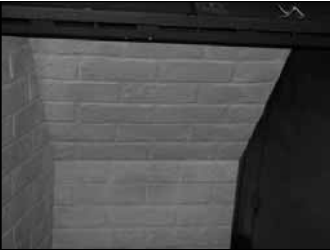
Figure 14.4 Install Upper Back Refractory
